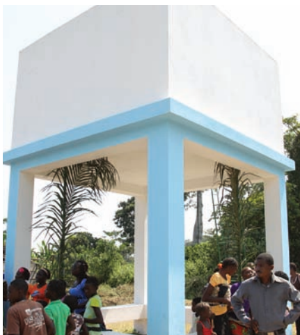
Water supply tank at the Mandarin Health Post
