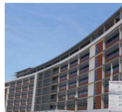
Chicala building in Luanda, new headquarters of CABGOC
